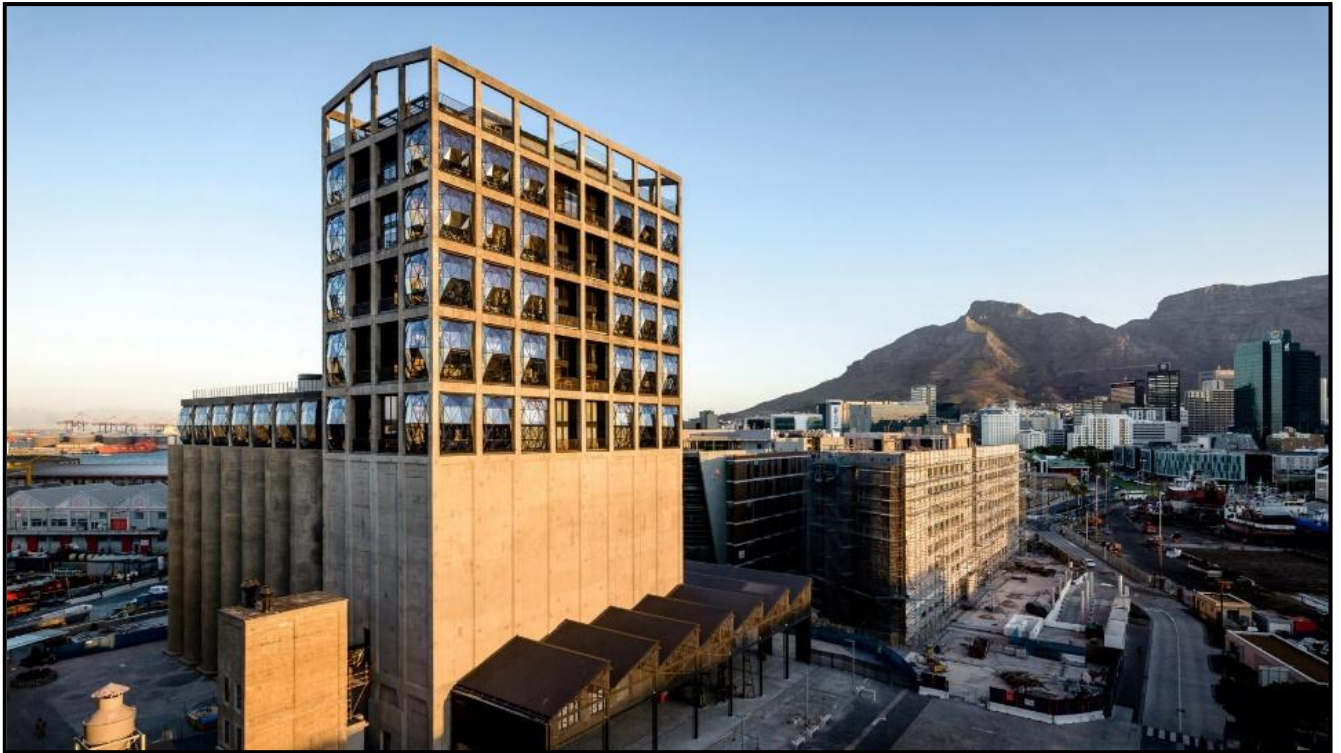
FIGURE 8a: Exterior view of the Museum of Contemporary Art Africa (Zeitz MOCAA) , Heatherwick Studios, Van Der Merwe Miszewski (VDMMA) and Rick Brown Associates (RBA), Cape Town, 2017.
