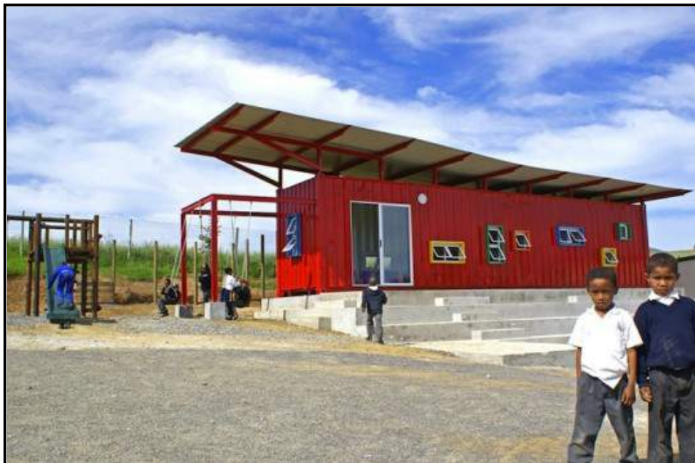
FIGURE 8b: Tsai Design, initially conceptualised by 15-year-old Marshaam Brink, Vissershok Container Classroom project , Du Noon township, South Africa, recycled containers, concrete, glass and polystyrene, 2012.
