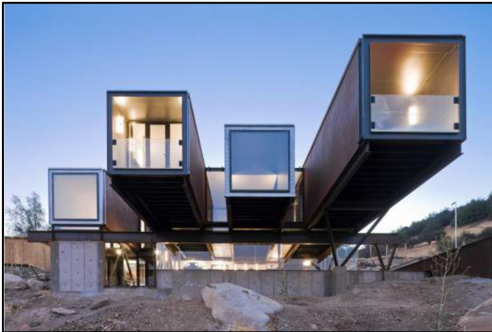
FIGURE 8a: Sebastián Irarrázaval, Caterpillar House , a shipping container-based family residence overlooking the Andes Mountain, Chile. The house comprises 12 shipping containers which provide bedrooms, living quarters and a swimming pool, 2012.
