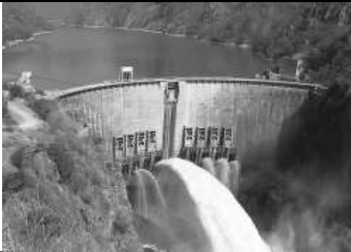
Cahora Bassa Dam
