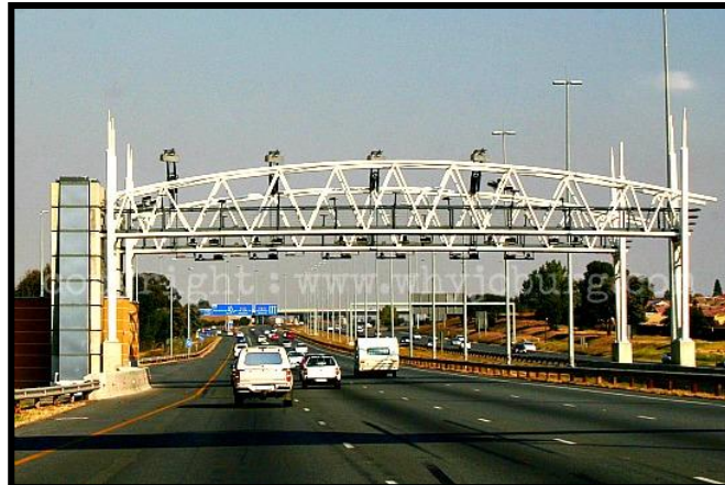
Image of an e-toll gantry on the N1 freeway in Gauteng
